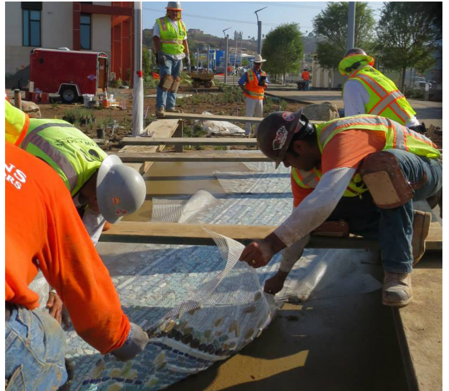
2. Crews laying mosaic on wet monolithic concrete.
