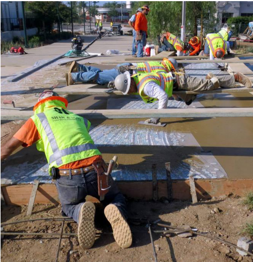
3. Troweling into the concrete.
